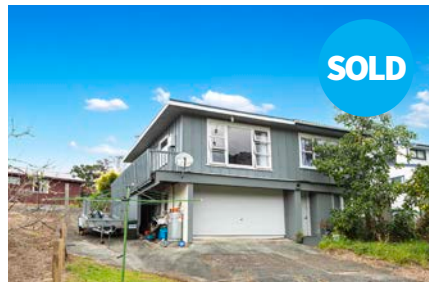
964 Whangarei Heads Road, Parua Bay
